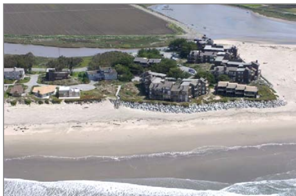
Figure 5-12: Pajaro Dunes Pelican Point Condominiums Source: California Coastal Records Project.
